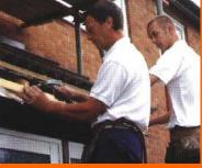
A new treated timber fascia support is attached to the rafters to ensure that uPVC is completely straight when installed.
