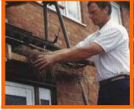
The roofline had only provided limited protection to the roof and a bird's nest was discovered. Installers remove debris from the roof.
