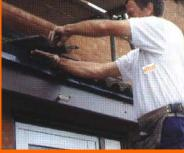
The tiles are put carefully back into place. The bird comb, which is positioned under the tile, will prevent any birds or other vermin making your roof their home.
