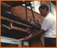
Worn and rotten timber fascias and soffits are removed along with all existing roofline to ensure there is no damage to the property.
