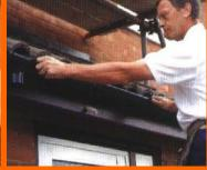
After the gutter brackets are fixed to the fascia board using stainless steel screws, the gutter is clipped in to the brackets.
