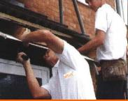
The rafter ends are thoroughly checked for rotten timber before any new material is installed.
