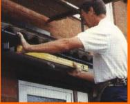
The installers use a spirit level to guarantee an adequate slant on the gutter. The fall on the gutter will allow rainwater to flow smoothly into downpipes.
