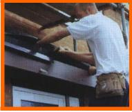
The Over Fascia Ventilation and Eaves Protection is put into position. The customer will not have to worry about rotten rafters or pools of water collecting in the roof.
