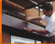
The uPVC fascia board is fixed using stainless steel nails. These do not rust and have colour matched heads and virtually invisible.
